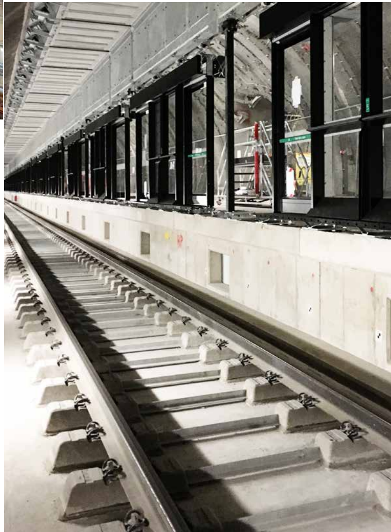
▼ Bond Street Station in der Bauphase.
