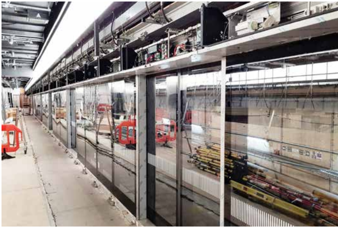
▲ Canary Wharf Station in der Bauphase.
